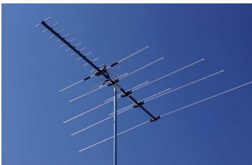
This type of antenna is no longer needed in this area. This antenna was used in the analogue television days. It could now be causing problems with digital reception by picking up random interfering signals and degrading signal quality
